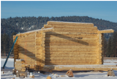
Construction of the first cabin
